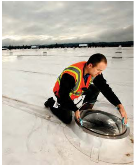
The solar tubes atop the Lowe's Flatbed Distribution Center in Centralia, Wash., can provide sufficient lighting even on cloudy days.
