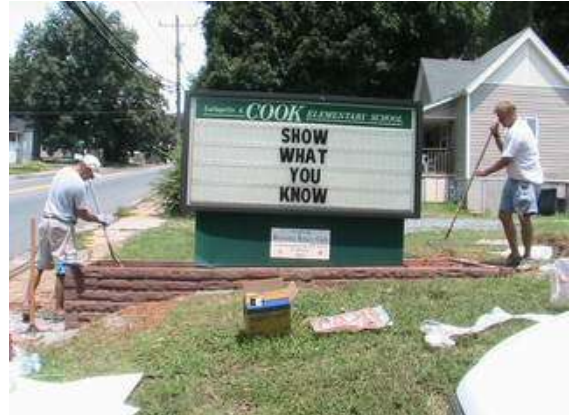
Lowe’s Heroes spent three months revitalizing Cook Elementary School, replacing broken windows and brightening up the 55-year-old campus’ courtyards and classrooms.
