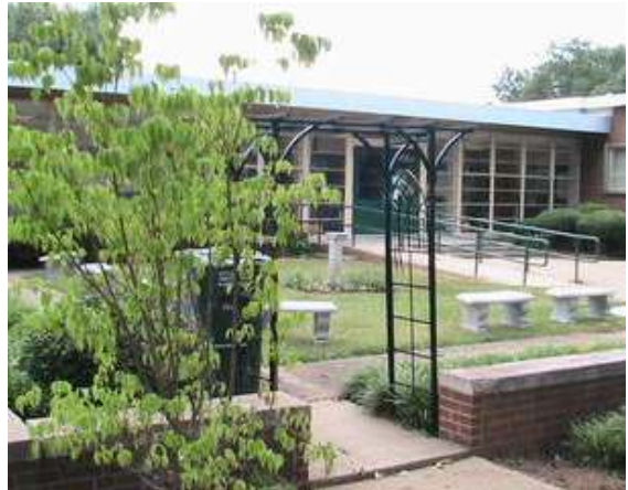
Lowe's Heroes spent three months revitalizing Cook Elementary School, replacing broken windows and brightening up the 55-year-old campus' courtyards and classrooms.
